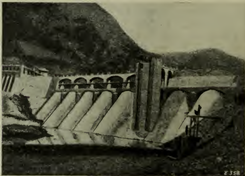
VIEW SHOWING FINISHED UPSTREAM SIDE OF DAM.
